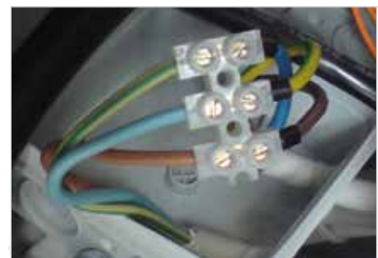
Fig. 7: The N and PE have been interchanged here
